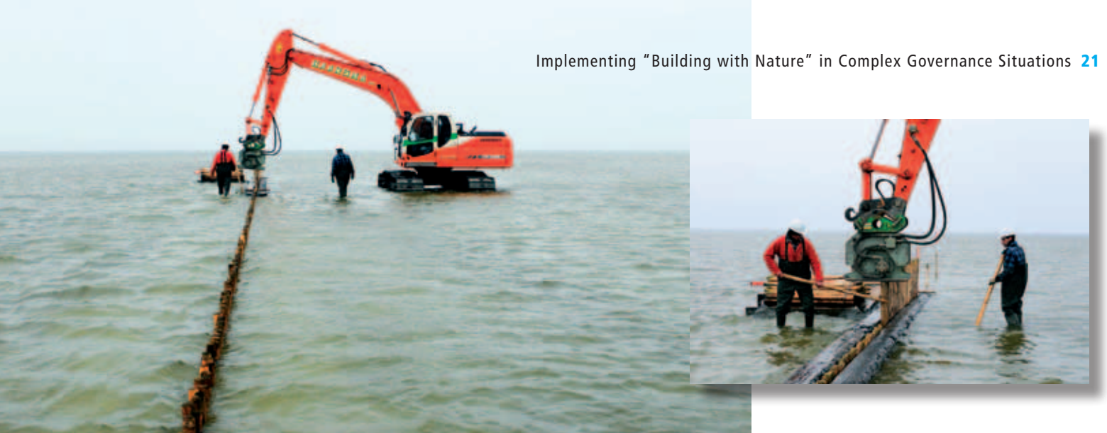
Figure 3. As part of the pilot study on the Frisian IJsselmeer coast, a semi-permeable row of poles was constructed. This row must mitigate wave energy so that sand can deposit at the location of the Sand Engine. Insert, close-up of the poles being placed.
