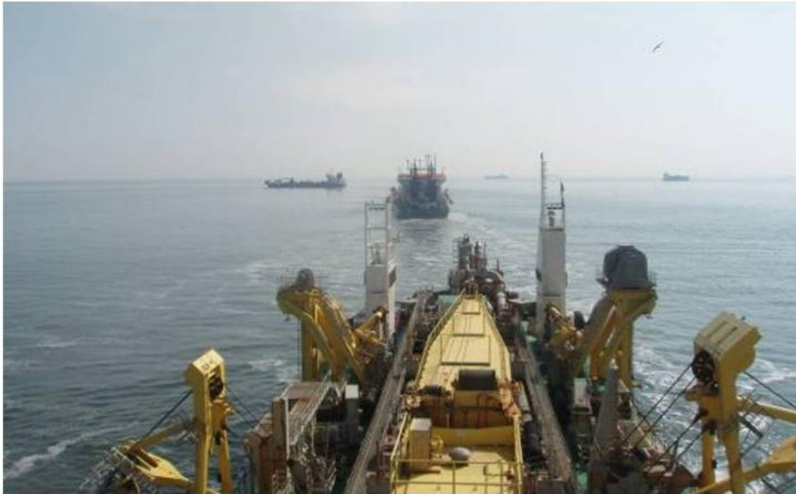
Figure 4-2: Dredging ships creating the parallel sand ridge that lies to the left of the ship.
